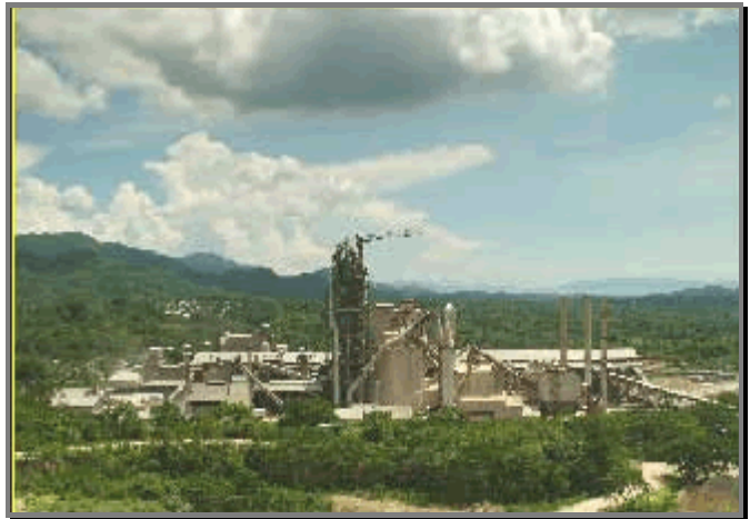
RCC Batangas Plant has received international certifications. QMS: ISO 9001: 2000, EMS: ISO 14001: 2004, HSMS: OSHAS 18001: 2007
