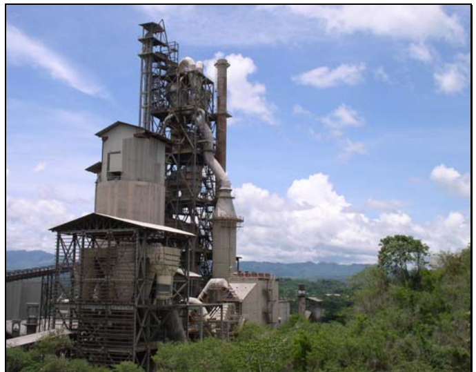
RCC Teresa Plant has received international certifications. QMS: ISO 9001: 2000, EMS: ISO 14001: 2004, HSMS: OSHAS 18001: 2007
